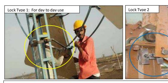
The encircled portion shows two different types of lock being incorporated in the windmill
