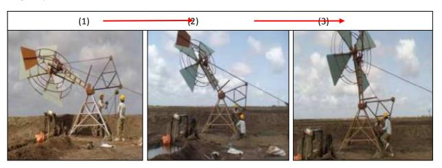
Using this, speeds up the installation process and it also reduces the risk factor, which was earlier associated with the installation process. This also requires less labor to erect the windmill.
